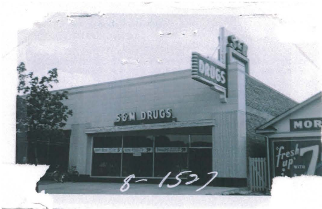
Historic Photo - 416 E 900 S – West End
