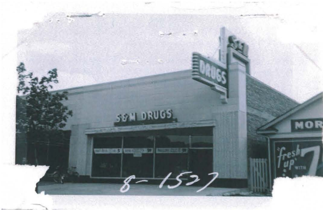
Historic Photo - 416 E 900 S – West End
